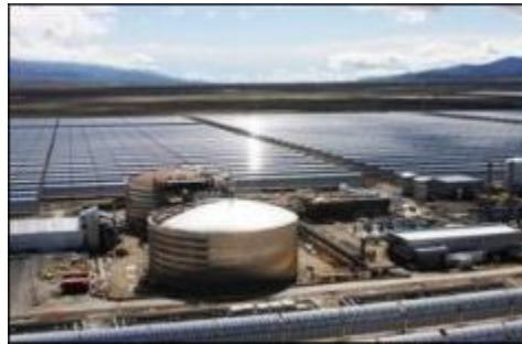
Molten salt storage, Andasol power plant, Spain: up to 400/565\text{ }^{\circ}\text{C}
