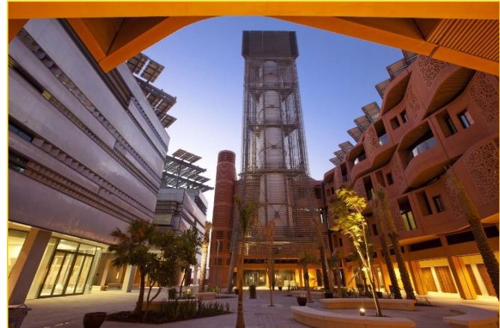
EnergyNest AS Office, Masdar City, UAE
