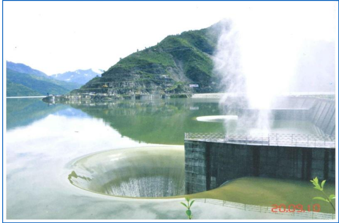
Tehri PSP Project - India
