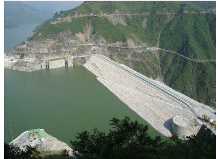
Tehri PSP Project - India
