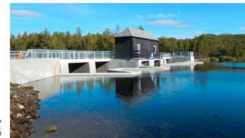
Dam in the Tasse reservoir. Photo: CLB
