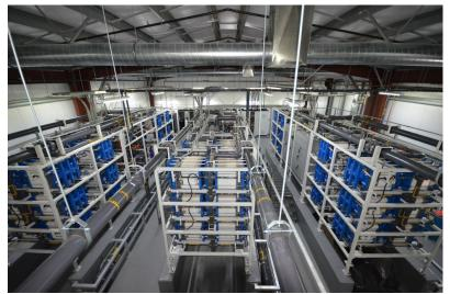
Flow batteries: Gills Onions, California: 600kW, 3.6 MWh
