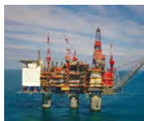
Electricity for oil and gas production
