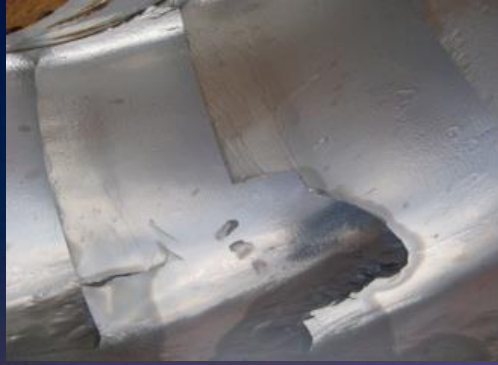
23 MW*2 Francis runner at Chawa Power plant, Chile
