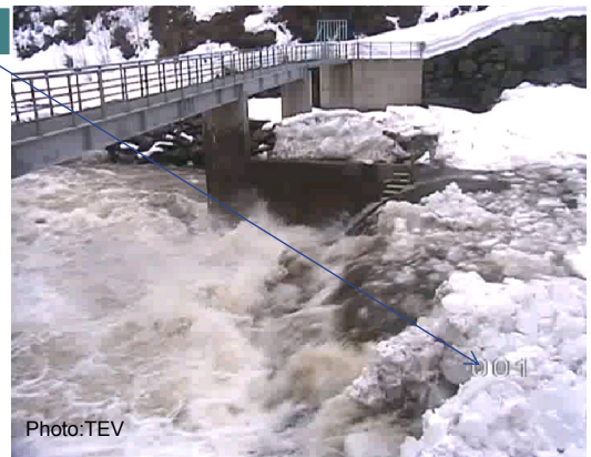
Intake Blockage
