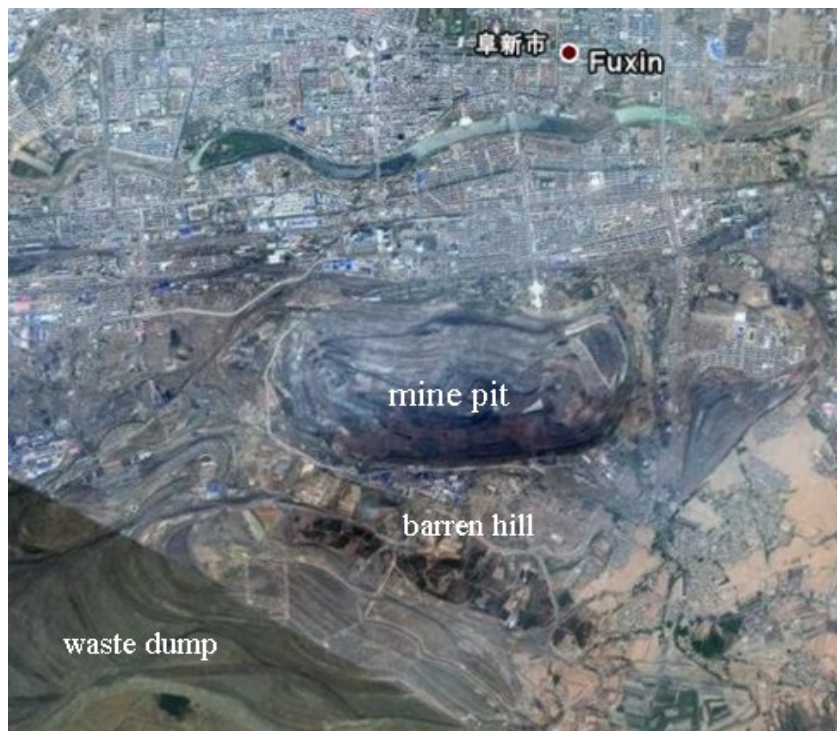
Figure1 satellite image of Haizhou open-pit mine
