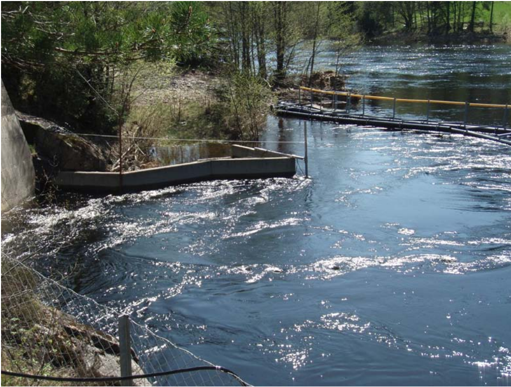
Figure 5-4. The photos shows the intake reservoir and the actual inlet to Laudal hydropower plant to the left.
